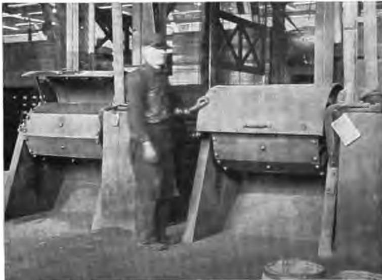
Fig. 2. Tumbler Guards, raised and lowered.*
